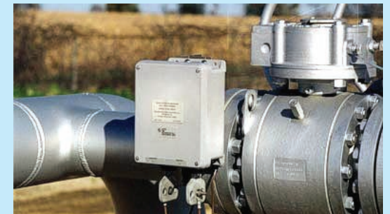
Polarization Cell Replacement (PCR)
